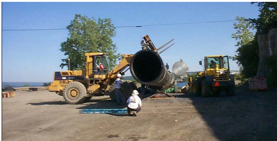
Figure 29. Loading pipe (63”) into fusion machine with front end loader.
