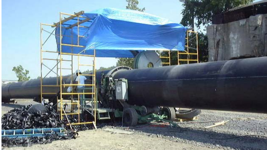
Figure 28. Fusion machine set up to fuse 63” HDPE pipe.
