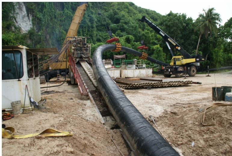
Figure 43. Example of HDPE pipe being placed via Horizontal Directional Drilling.
