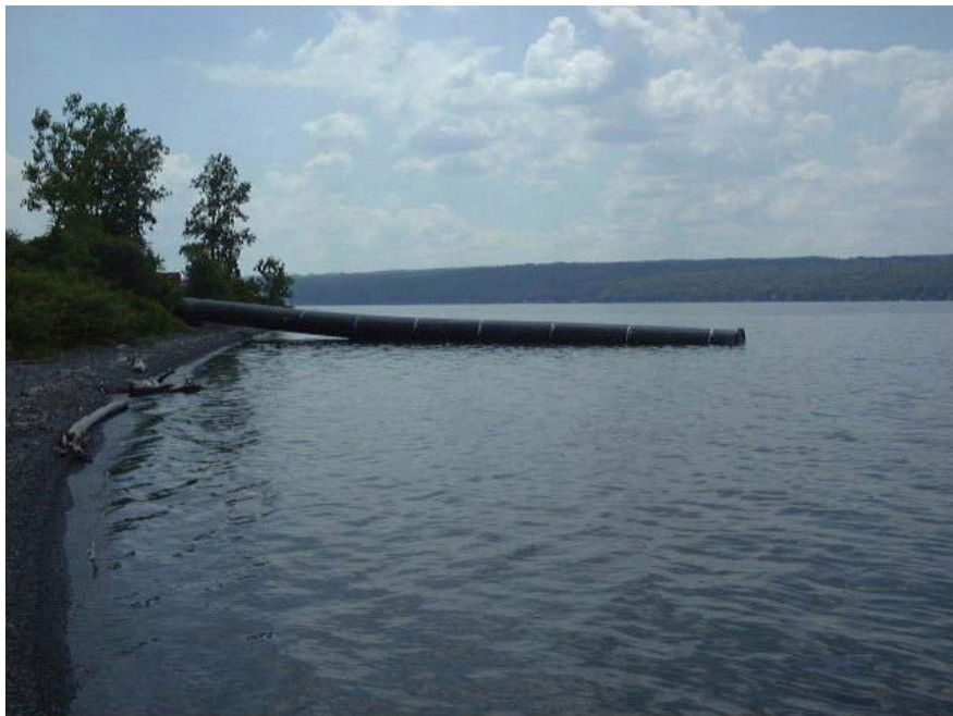
Figure 31. Fused pipe (63") entering the water.
