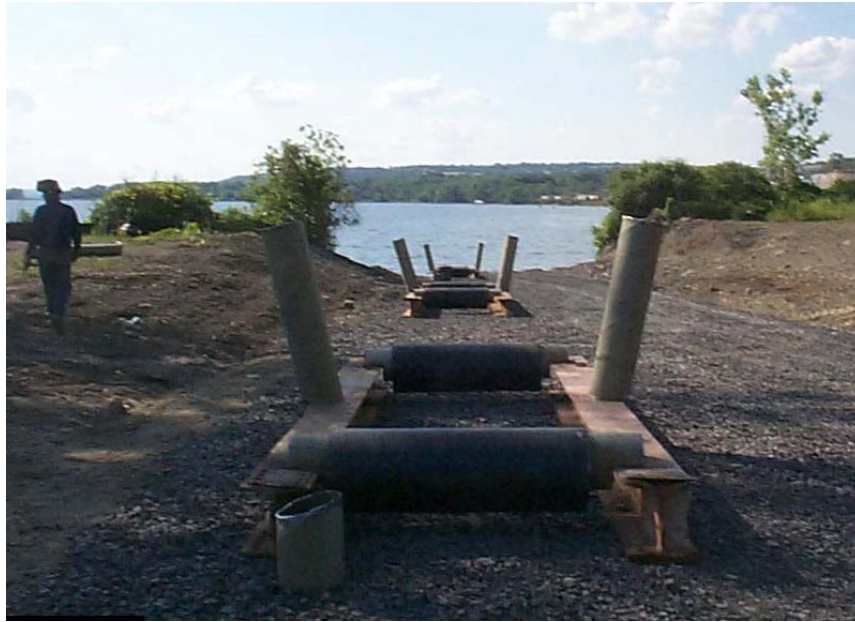
Figure 30. Roller beds used to move fused pipe down to the water.
