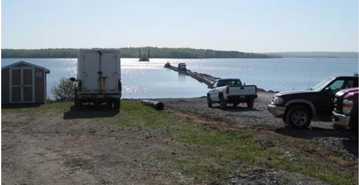
Figure 7. Example of temporary causeway built for HDPE pipeline deployment at the Northern Pulp Mill staging site. Photo from 2009 courtesy of Northern Pulp.
