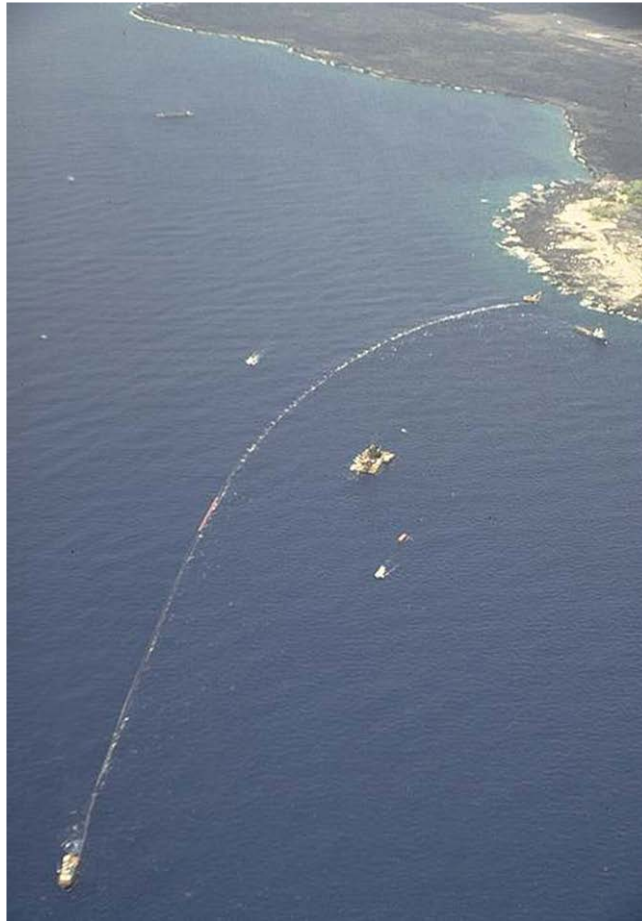
Figure 38. Deep water pipe deployment – maneuvering to counter cross-currents.
