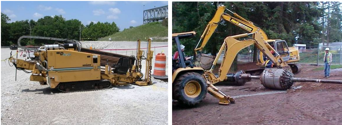
Figure 41. HDD drill rig (left) and reaming head (right).
