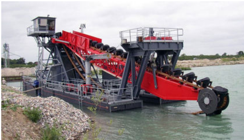
Figure 13. Conventional excavation dredging
