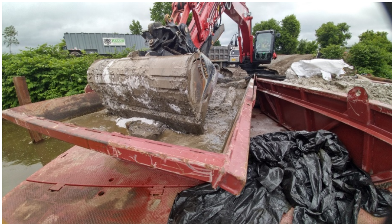
Figure 15. A clamshell excavator placing spoils in a dredge box
