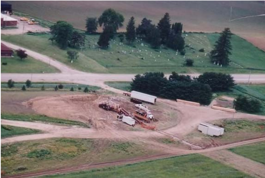
Figure 42. Aerial view of HDD in progress.
